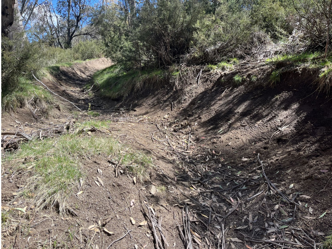
Figure 11: Example of trail quality of berm on steep section of Cannonball trail within the native vegetation post winter. The fallen leaf litter/debris protects the trail tread from erosion. Evident erosion is better managed through natural features vs treeless disturbed ski slopes. Photo taken 10 October 2023.
